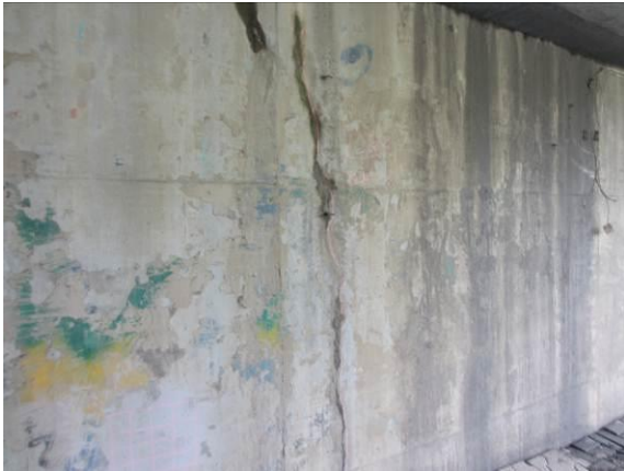
图3.2.2-2 Y-3#桥台前墙竖向裂缝，距左侧 5.4m，通长，d=0.46mm
