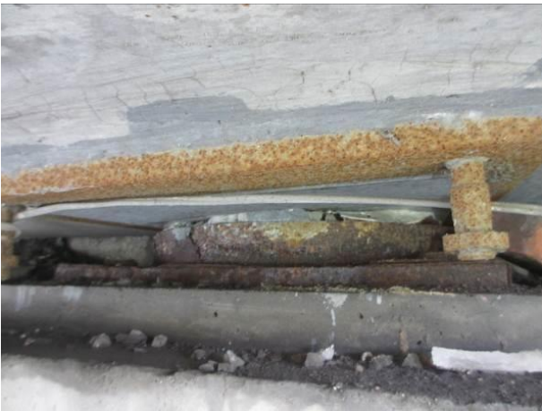
图3.2.2-5 Y-3-1 支座钢板锈蚀
