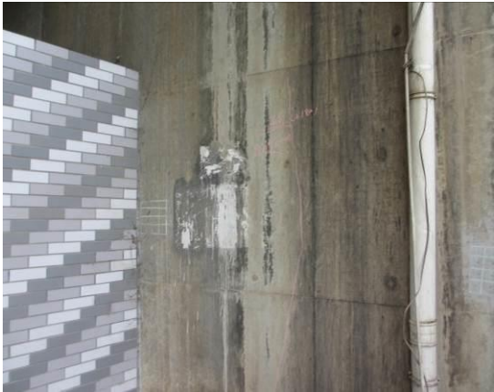
图 3.2.1-1 Z-0#桥台前墙竖向裂缝，距左侧 2.4m，通长，d=0.34mm
